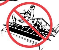
**⚠ DANGER** Do not walk on trusses or gable end frames lying flat, they do not have the structural strength to support a worker safely while oriented flat.
