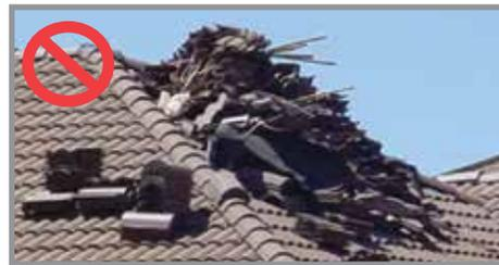
**DON'T** pile cut-off tile and/or other construction waste on trusses.
