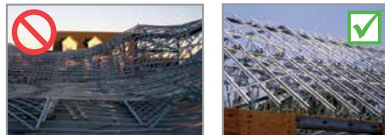
**NOTICE** Lateral restraint is NOT adequate without diagonal bracing.
