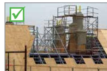
Install all permanent building stability bracing immediately.
