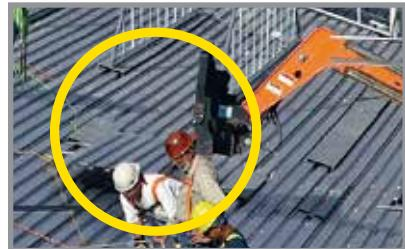
**DO** leave construction materials on lifting equipment until installation, if possible.
