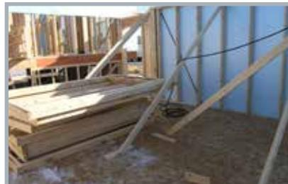
**Step 10:** Install the upper top plates at all locations that have been omitted for installation purposes.
