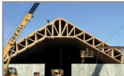
trusses can be installed safely and efficiently but require more detailed safety and handling measures than shorter span trusses.
